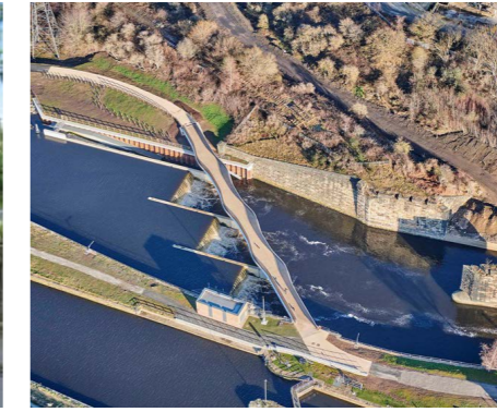
Knostrup Weir, Leeds | Flood Management Provides three new pneumatically moveable weirs that can be lowered to let floodwater discharge quickly downstream.
